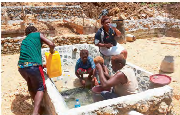
Water Project: School of Allied Signs, Namatanai, 2016
